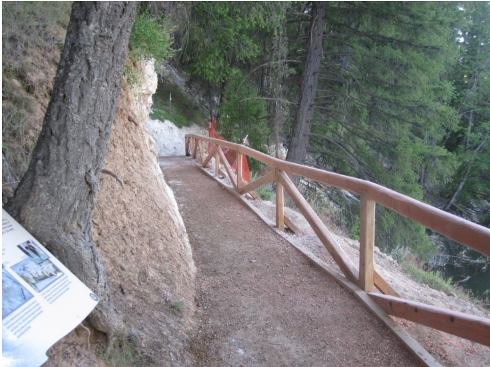
Photo 18.3 - Railing with Buried Post Sills
